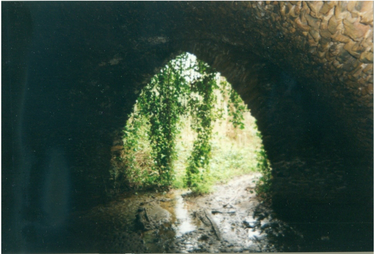
Inside-out from Mother Ludlum's showing water flow; photo by Ken Parsons
