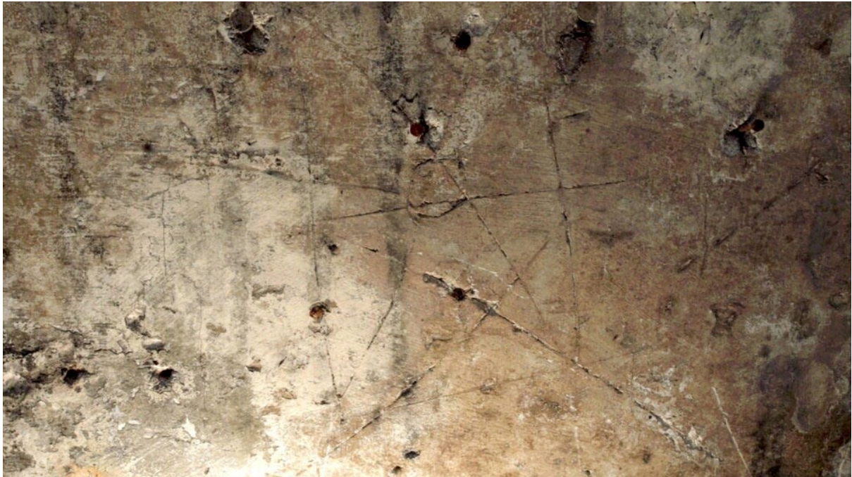
The 5 pointed star that was drawn into the wet plaster when the house was built in the 1730s
