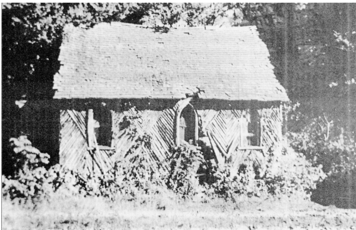
THE CONGREGATIONAL CHAPEL IN EASHING. This shows the chapel in its original setting before removal and restoration. It was built by the Petotress family the Congregational owners of Eashing paper mills.
